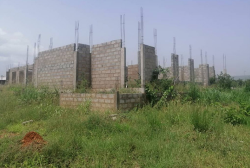
GETFund Project: Library and Laboratory Block
